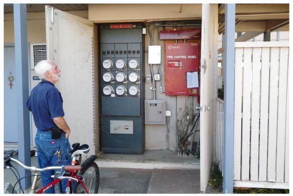
Photo No. 18 Utility cabinet containing electrical meters, telephone lines, and fire control system on the east side of Building 5100
