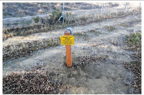
Photo No. 23 Sign indicating a buried natural gas pipeline in the western portion of the Site
